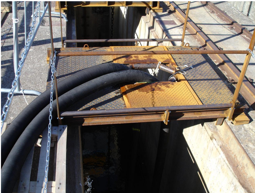
Figure 2-13 Hoses which directed eels to the desired release points.
